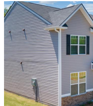
Foundation wall is only located on the front façade
