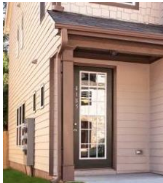
Foundation wall missing / insufficient height on the side
