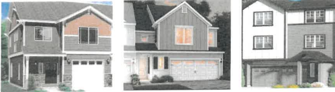
Brick or stone is only partially used or is not used at all as the required exterior finish, and carriage-style garage doors are not used. In addition, required elements over the projecting garages (left and middle examples) are missing.
