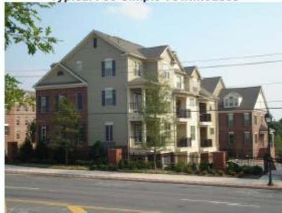
Apartments with Good Articulation of Buildings
