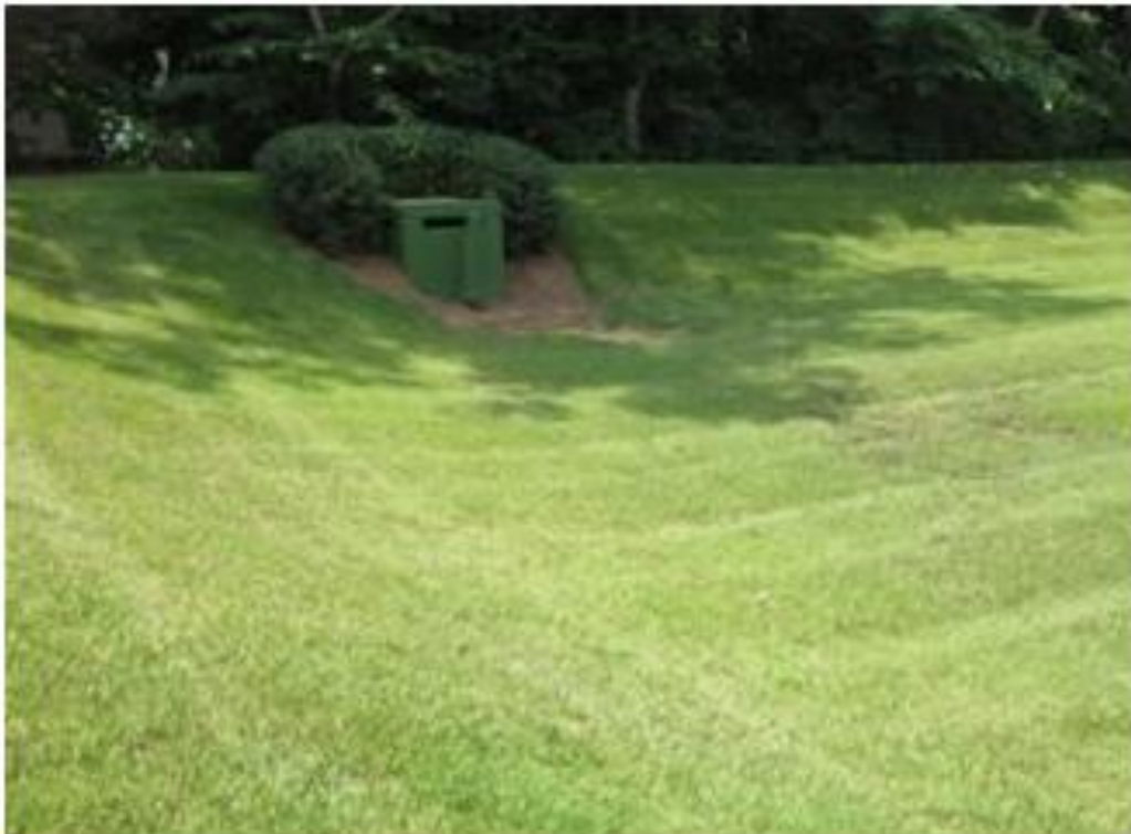
Dry Detention Pond Properly Maintained
