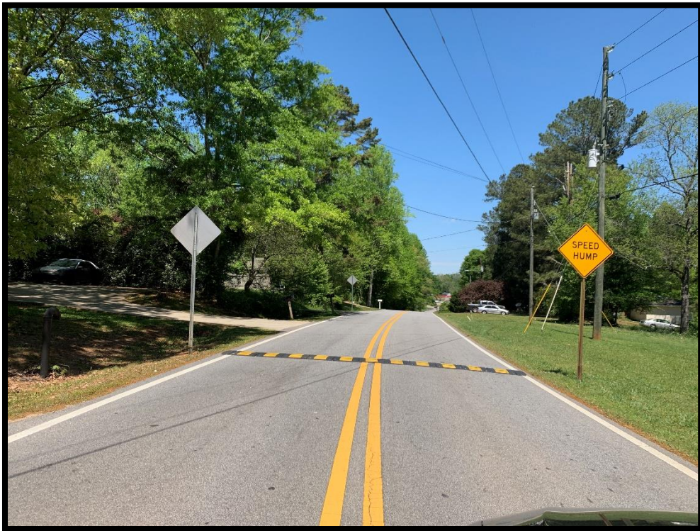
Photograph 3 – Speed Bump on Mulberry Street
