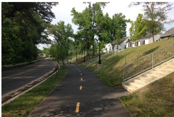
The berm and staircase limit access to homes without having a fence
