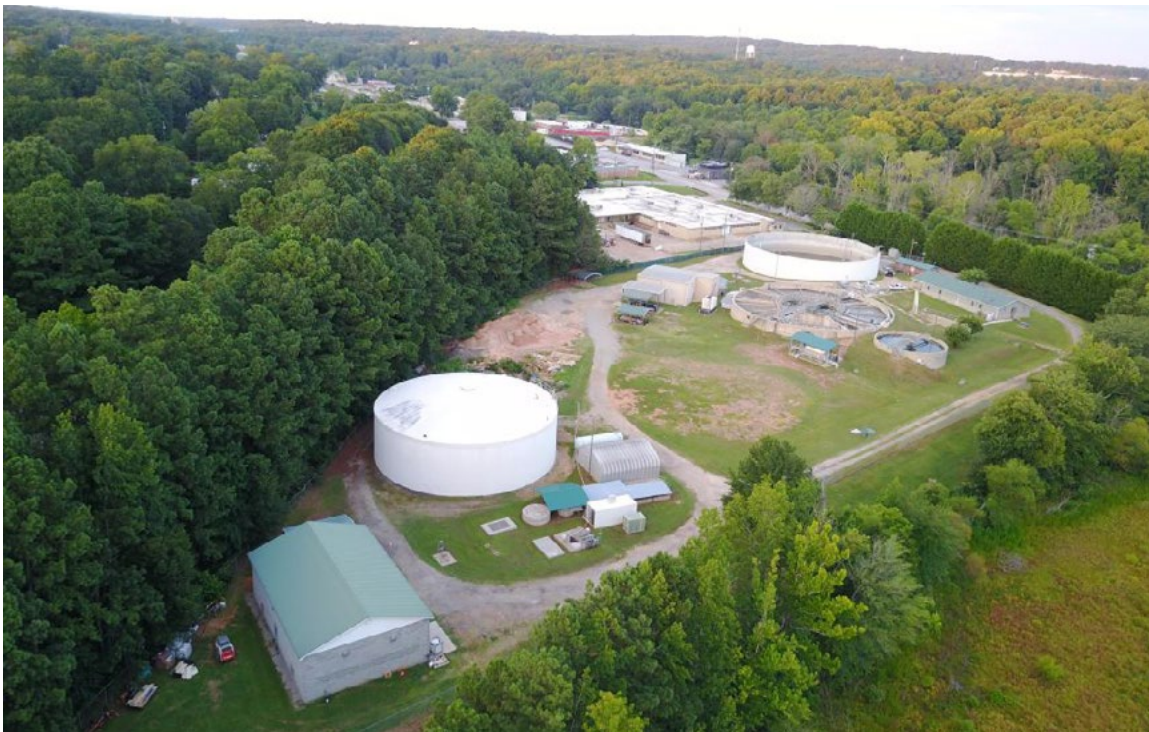
Figure 6 - Flowery Branch Water Reclamation Facility
