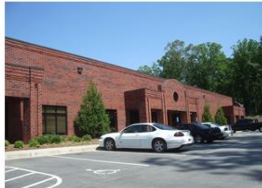
All Brick, Articulated Building Façade
