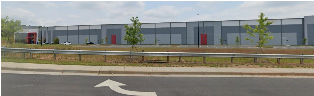
Tilt up modular concrete wall building Thurmon Tanner Road
