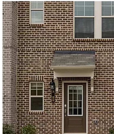
Shingled roof over front stoop
