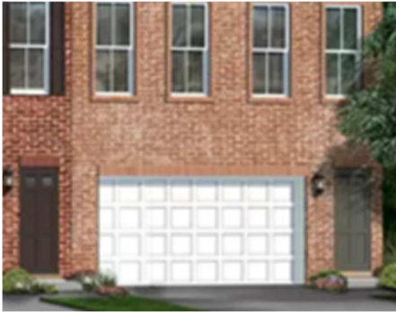
Garage is not recessed, and no projecting element is provided over the garage
