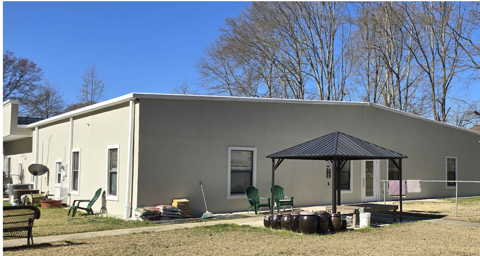
EXISTING BUILDING VIEW(REAR)
